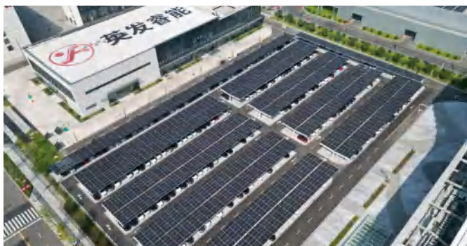
▲ A PV Power Station of Yingfa Deyao
